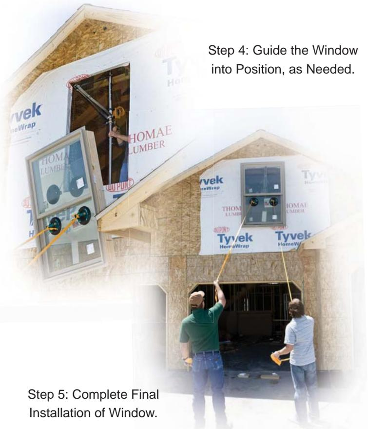
Step 4: Guide the Window into Position, as Needed.
